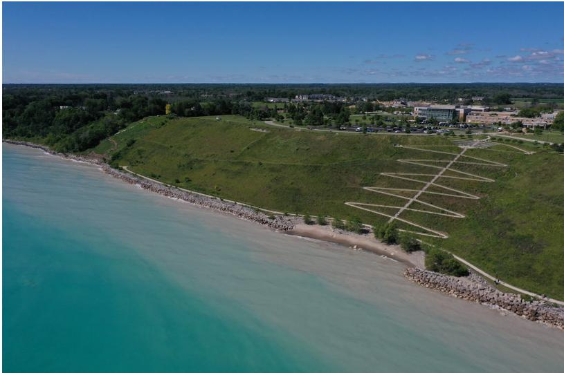
*In 2007, the Concordia University Wisconsin, in Mequon, Wis., finished fortifying a 130-foot bluff and building a 2,700-foot-long rock wall to buffer waves. The \$12 million project was among the largest built along Lake Michigan in Wisconsin. The project has accelerated erosion on downstream properties from around 9 inches to more than 7 feet per year. (Coburn Dukehart / Wisconsin Watch)*
